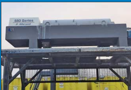
550-Series Alfa-Laval Platform Mounted Centrifuge w/ Yaskawa & Square D Altistart Controls
